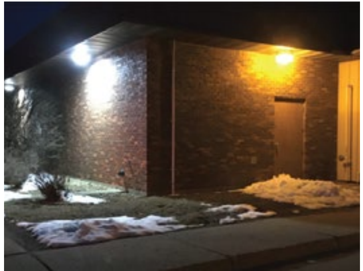
Old lighting (right) versus white LED lighting (left) of Federated Rural Electric's Jackson office. Federated Rural Electric offers LED lighting rebates to help offset installation costs to improve lighting and decrease electric bills.
